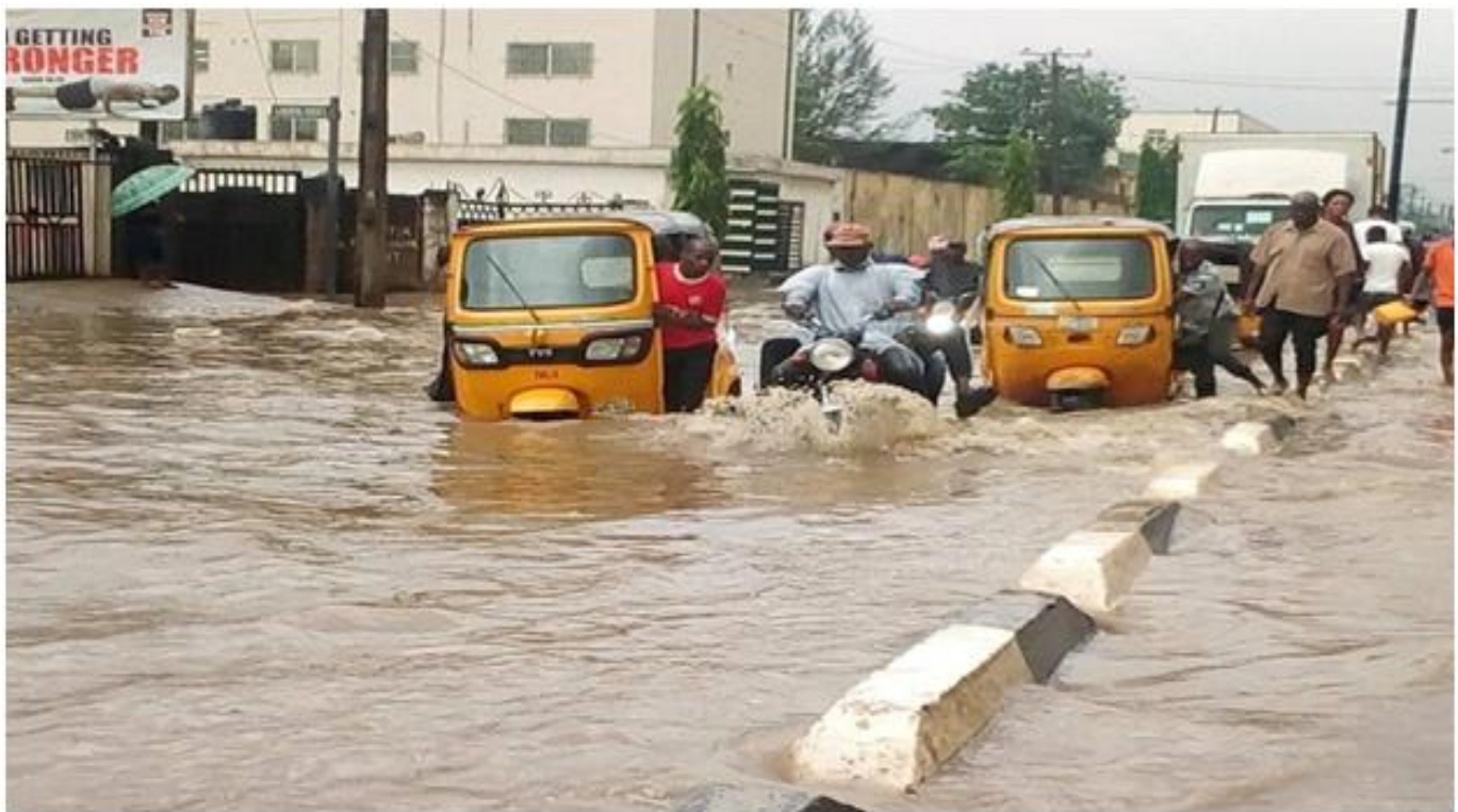
Figure 1: Flooded Road situation in Makurdi (Source: independent.ng)
